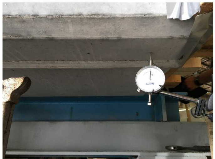
Figure 8: Front view of crack after failure load
